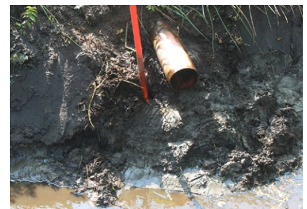
Drainage pipe in a newly maintained ditch.
